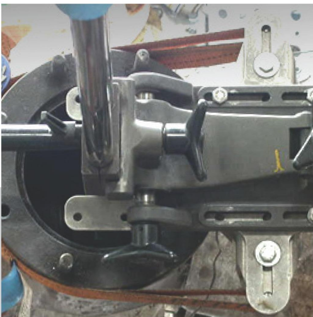
*대구열병합발전소 1500# 8" Gate Valve Seat Lapping SL-2 작업모습
